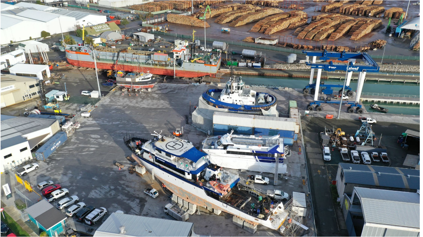
Aerial view of the Calwell Marine Maintenance Facility. Credit: Tim Cuff
