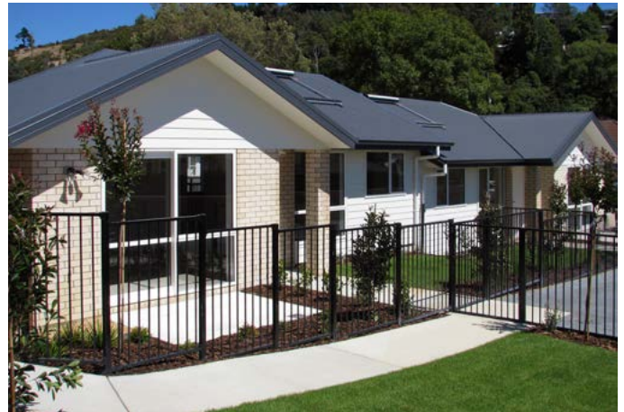
Kawai Street South housing. Credit: Nelson Tasman Social Housing Trust
