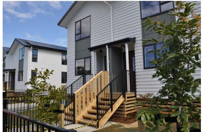
Totara Street housing. Credit: Nelson Tasman Social Housing Trust
